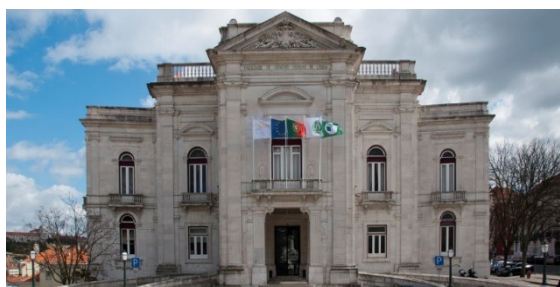
Figure 43 - Building S - Head Office
