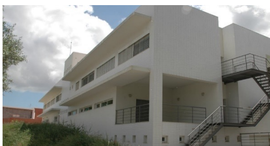
Figure 48 - School Building of the Pulido Valente Hospital
